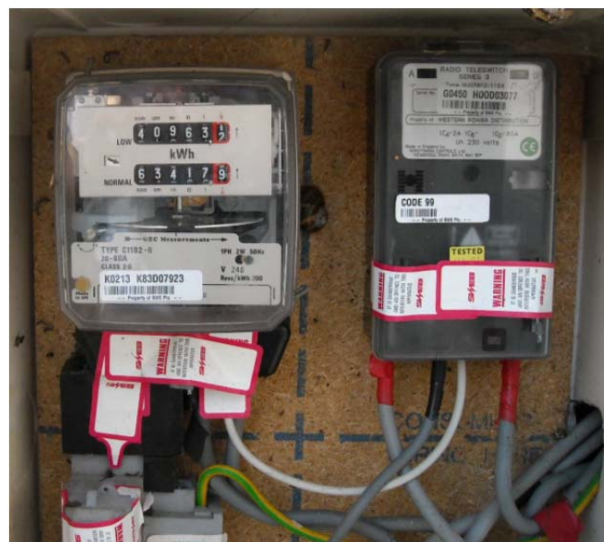
Figure 17. Analogue meter with two electricity readings for peak and off-peak tariffs
