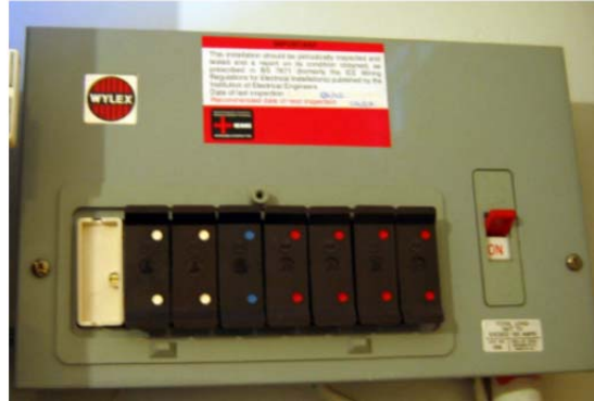
Figure 19. Older design consumer unit with rewirable fuses
